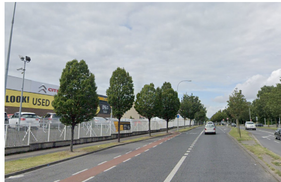
Image 11. Street planting of early mature fastigate hornbeam north of the Clearwater shopping centre.
